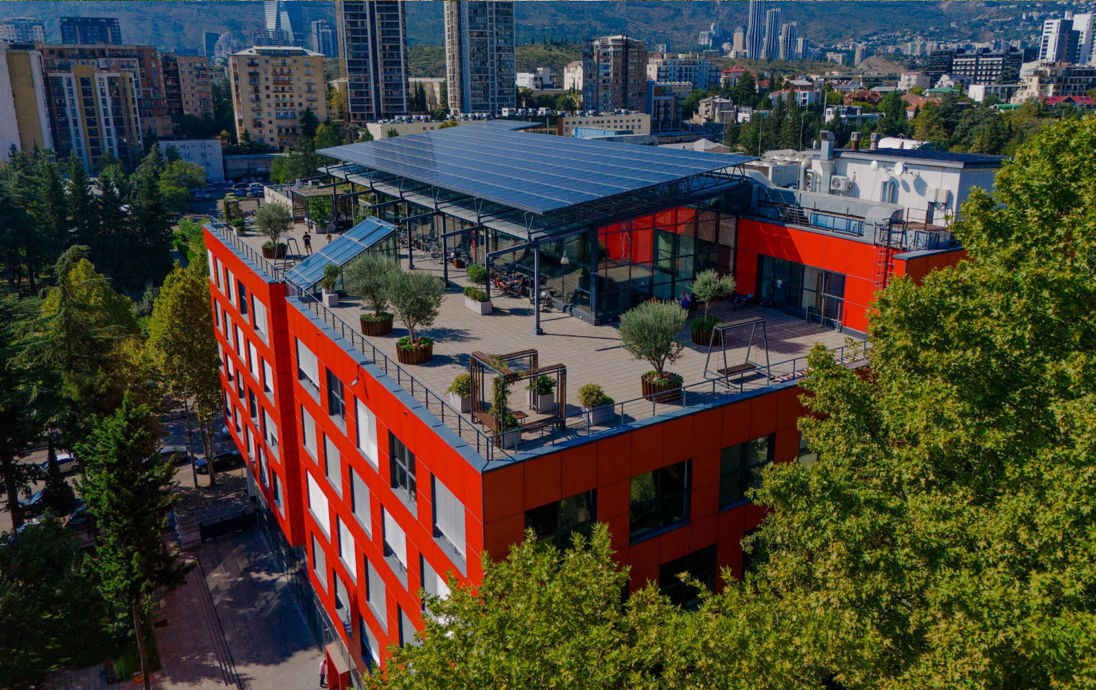
Above: Tri Sunca, electric power generation, transmission and distribution. Client of ProCredit Bank Bosnia and Herzegovina Below: Head office of ProCredit Bank Georgia in Tbilisi
